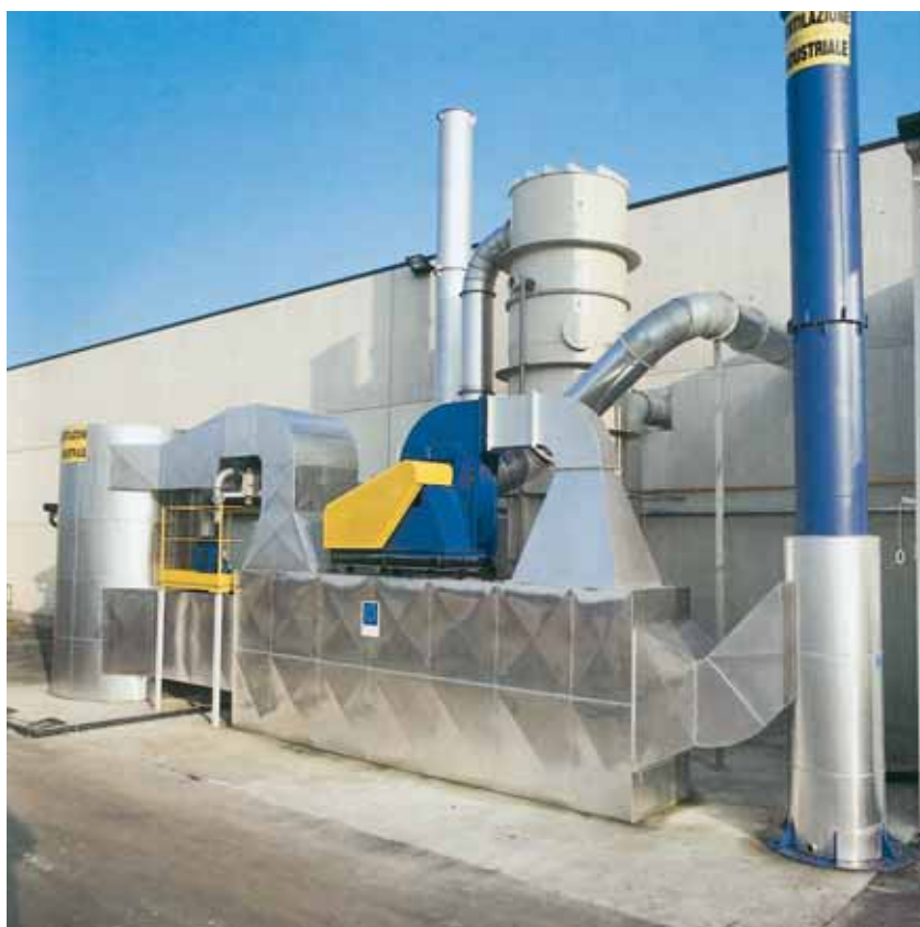
Catalytic combustion plant, 8000 Nm 3 /h, installed at a company sensitizing aluminium photographic sheets.
